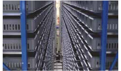
Rail dependent storage and retrieval equipment
